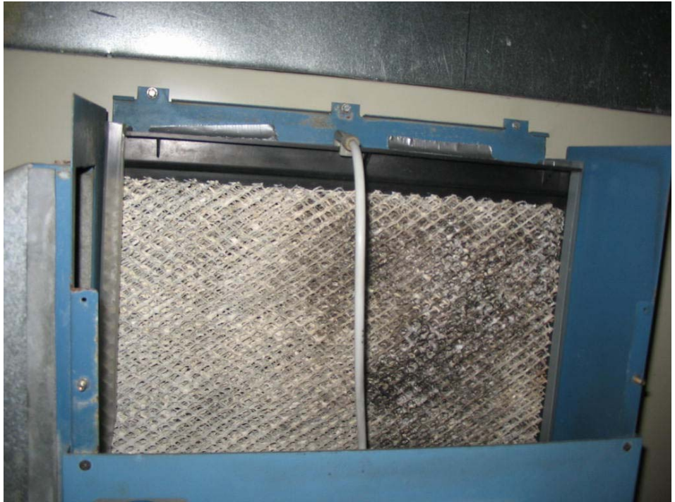
The humidifier pad is dirty. Clean the unit, and replace pad.
