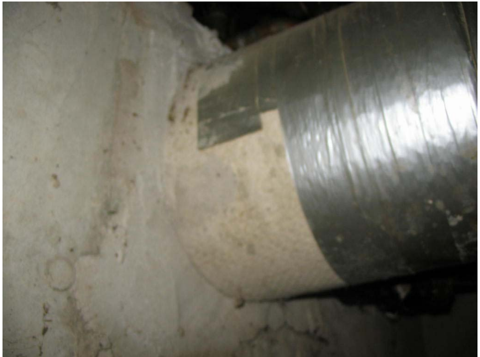
There is white material on/in some of the heating ducts/vent pipes. It is possible that this may contain asbestos. Unable to determine without laboratory analysis. Recommend further evaluation by a specialist.
