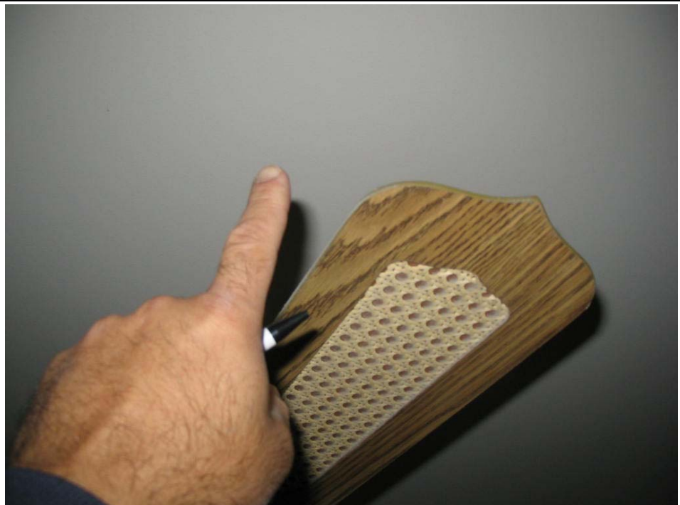
The ceiling fan(s) were too low. This poses a potential safety concern. Recommend removal.
